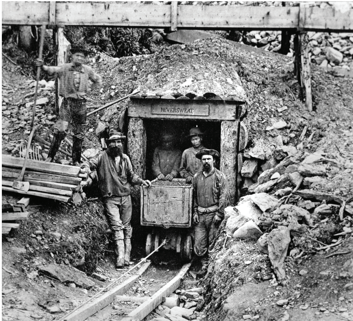
Shaft entrance of Neversweat Tunnel Co. Claim, Williams Creek – Frederick Dally ca. 1868, (BC Archives)
