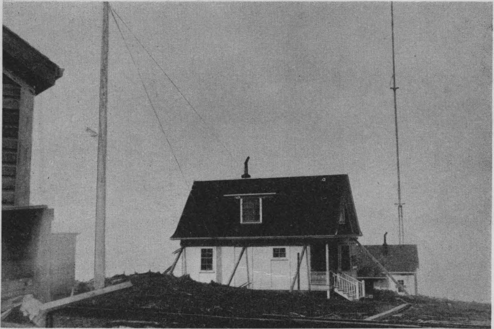
Fig. 4. Light-station and wireless buildings on Triangle Island, about 1915.
