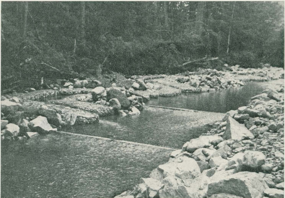
Improved spawning-channel provides optimum conditions of gravel, water velocity, and depth for spawning cutthroat trout, and side channels for rearing fry.
