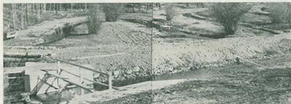
Eightythree Creek rainbow-trout spawning channel near Green Lake (Clinton district), showing stream-diversion structure in left foreground. Trees will be planted and natural ground cover encouraged to provide shade and cover for spawning trout.
