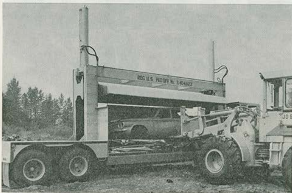
Derelict automobiles are compacted with this machine as part of the operations of Project S A M. The compacted vehicles are shipped to a shredding plant where the crushed scrap is converted into smelter feed.
