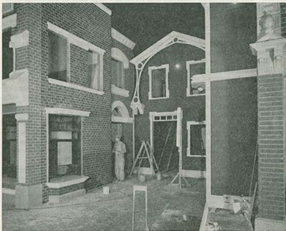
Project 70's street scene during the early stages of construction.
