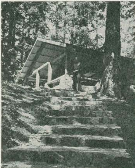
These stone steps were constructed at Little Qualicum Falls Provincial Park picnic-ground in an effort to reduce erosion caused by heavy visitor use.
