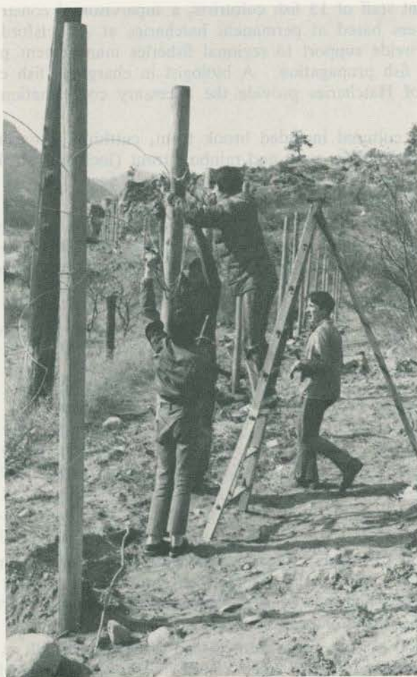
Sheep-proof fence being constructed near Vaseaux Lake to keep California bighorn sheep out of orchards in the area. The local Rod and Gun and Naturalists Clubs assisted in the project.
